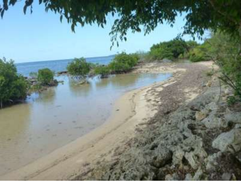
Coastline near Manuka Village where a failed seawall will be replaced with several short offshore breakwaters and mangrove replanting
