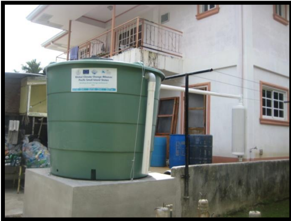
Client in Koror (Ngerbeched)
