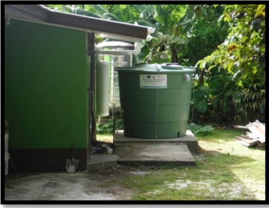
Client in Koror (Ngerbeched)
