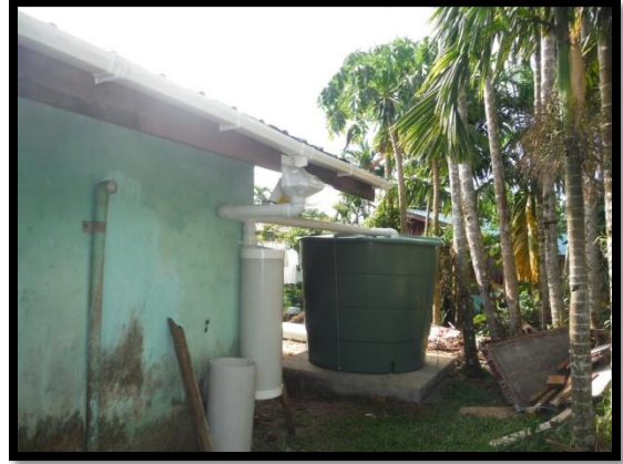
Client in Koror (Ngerbeched)
