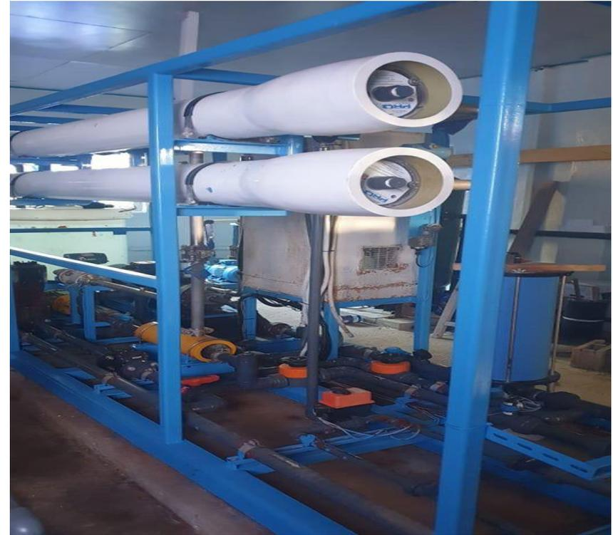
**Figure 1: 100m<sup>3</sup>/day Desalination Unit in Funafuti**
